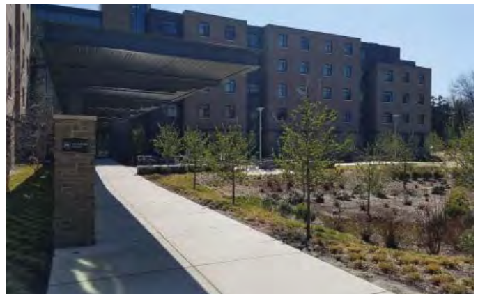
Penn State Abington Campus - Example of integrating stormwater management into the design of civic space at the entrance of a public/institutional building.
