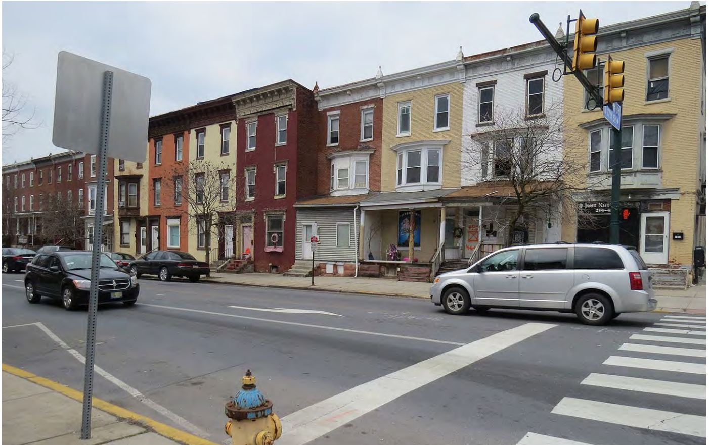
Market Street is relatively free of utility poles as the buildings are serviced from rear alleys.
